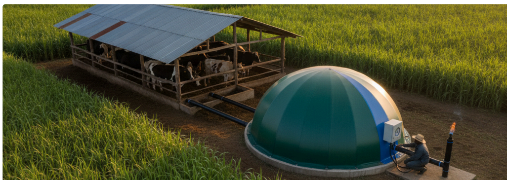
Figure 10: A properly sized biogas digester captures methane from manure, providing free cooking gas and electricity while producing odorless fertilizer for crops.
