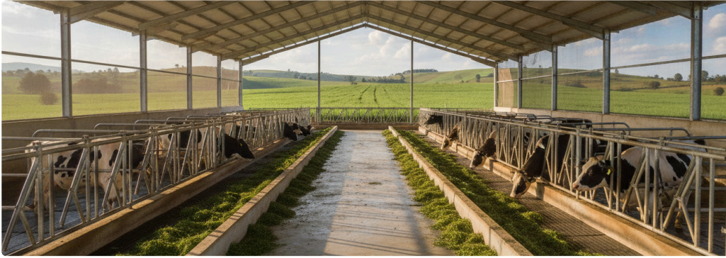
Figure 9: High-pitched roof design with continuous ridge opening creates natural convection that removes hot air and ammonia without electricity.
